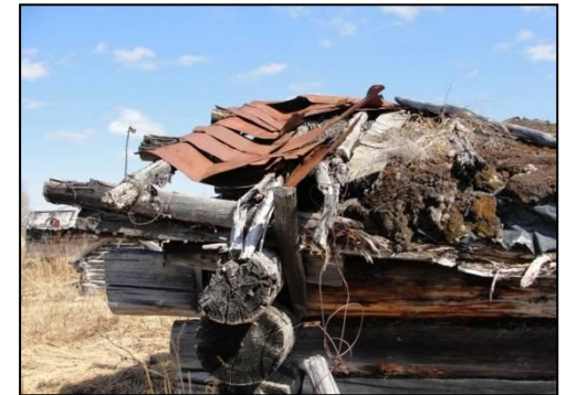
Roof with rain catchment drain made of Blazo cans, Telida Alaska
